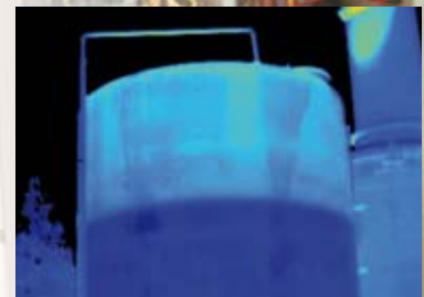
Tank level too low
